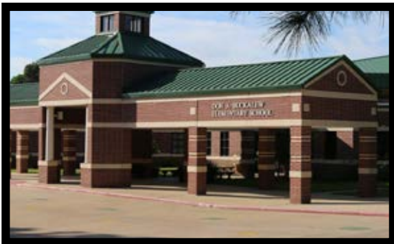
Buckalew Elementary School
