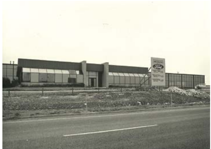
Remodeling the new Highway 6 Location
